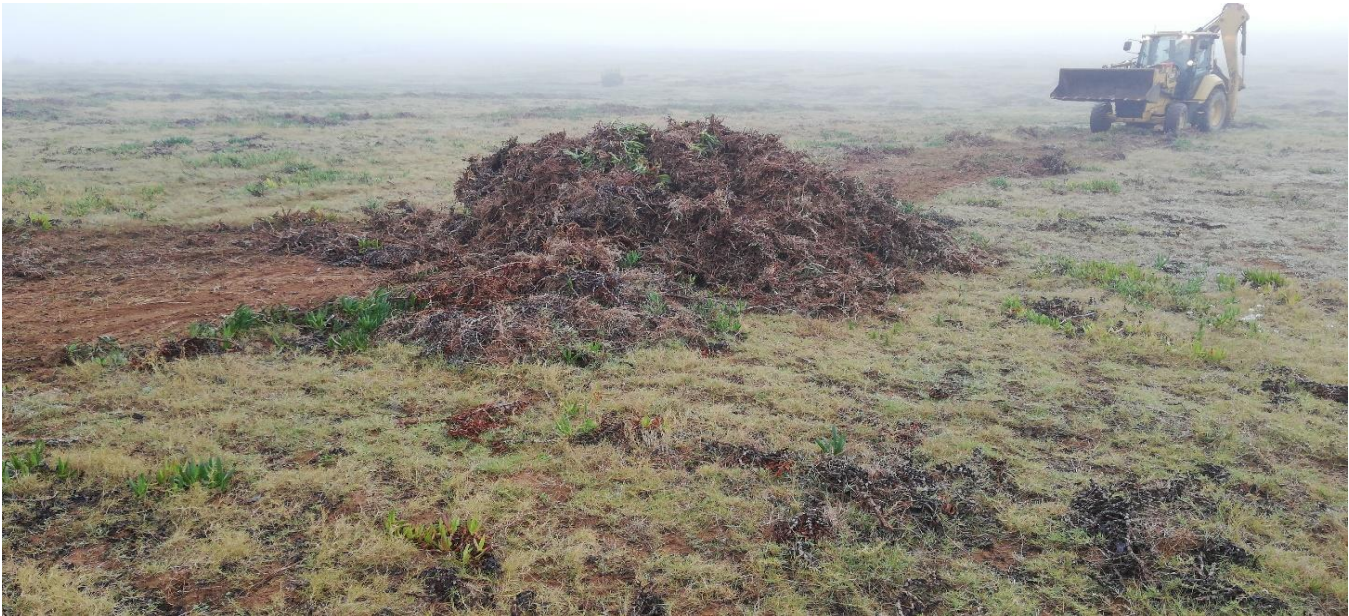
The digger loader pushing suurvy rows into heaps
