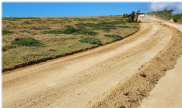
Grading activities of the main road
