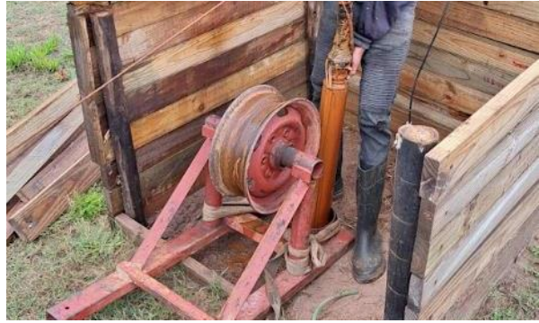
The red stains on the pump shows the presence of iron in the borehole water
