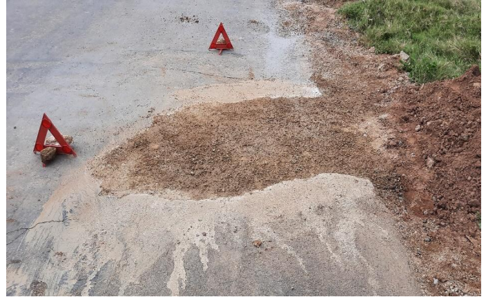
Pothole maintenance along the main road
