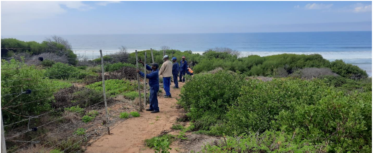
Above: Fencing team from Impi Wire Fencing replacing the Eastern fence.
