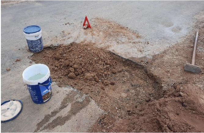
Pothole maintenance along the main road
