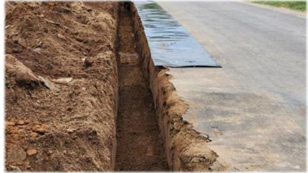
19 Jan 2023 – Excavation alongside the road with mole barrier being installed
