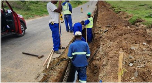
19 Jan 2023 – Excavation alongside the road with mole barrier being installed
