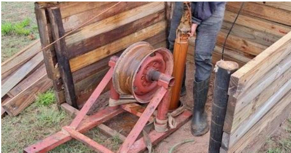
Re-adjustment of the borehole level and removing the pump for maintenance
