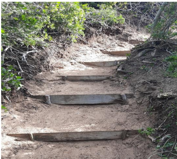
Repaired steps on red walking trail.
