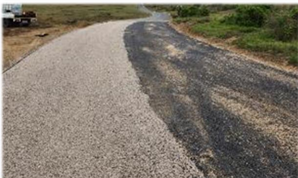
Working on the chip-and spray layer, with final product
