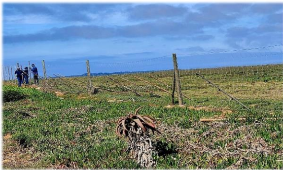
Western fence replacement in progress
