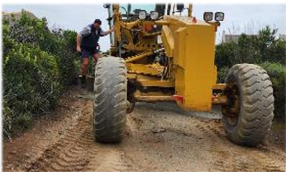
Placing of gravel with subsequent grading and compacting
