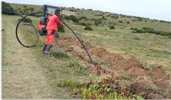
Placing the 50mm HDPE pipe
