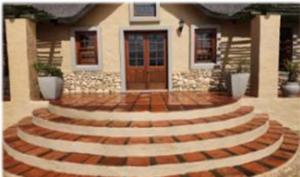
Upkeep at the office: linseed oil sealing at the stoep
