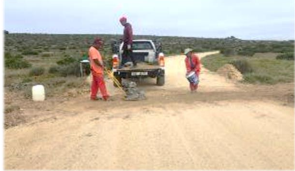
Compacting the trench at the crossing with the main road
